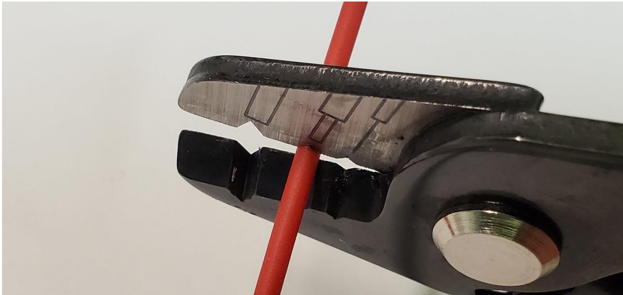
Figure 4. Remove Outer Jacket (be careful not to damage underlying LCP)
